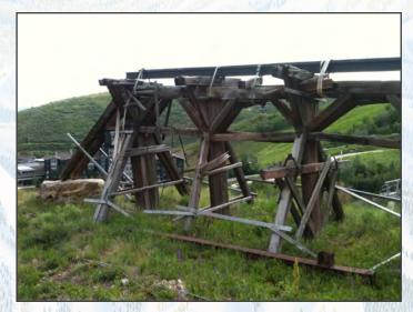
Aerial "tramway" systems were the direct precursors of modern ski chairlift technology and revolutionized mining. By replacing horse drawn wagons with overhead buckets, ore could be transported from Park City's mountains year round and avoid the inconvenience of huge snowpack. The counterweight held boxes of heavy rocks that anchored the King Con Tramway overhead cable. Remnants of the tram towers can be seen if you look on the hillside to the right as you ride up the Crescent Chairlift.
