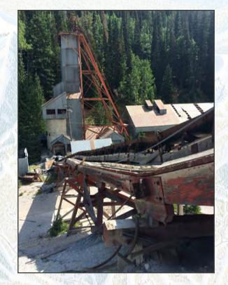
This enormous dump is the result of a futile exploration by the Silver King Coalition into barren ground. The conveyor took the waste rock from the shaft and tunnel system below and deposited it here on the dump.
