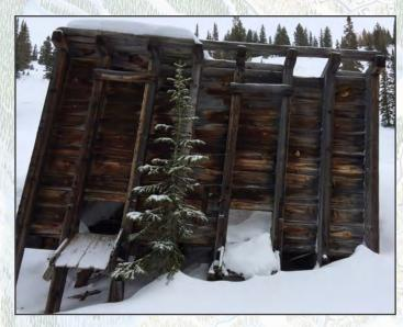
Ore was loaded into horse-drawn wagons through the ore bin chutes. It was a wild ride downhill to a mill in town. This structure is all that remains of a mining complex that consisted of three tunnels into The West Face of Jupiter Bowl.
