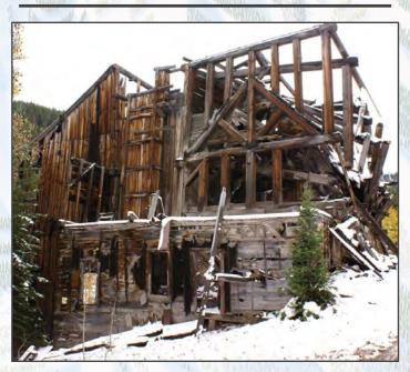
The California-Comstock stamp mill has been deteriorating since 1917 when it was last remodeled. It could process 150 tons of ore per day and was operated by very few men. Solon Spiro's Tunnel lies 1700-feet underneath this. It is connected underground to the Thaynes Shaft via the West End Tunnel where skiers used to ride the Skier Subway to alight at Thaynes Lift in the early days of Treasure Mountain Resort.
